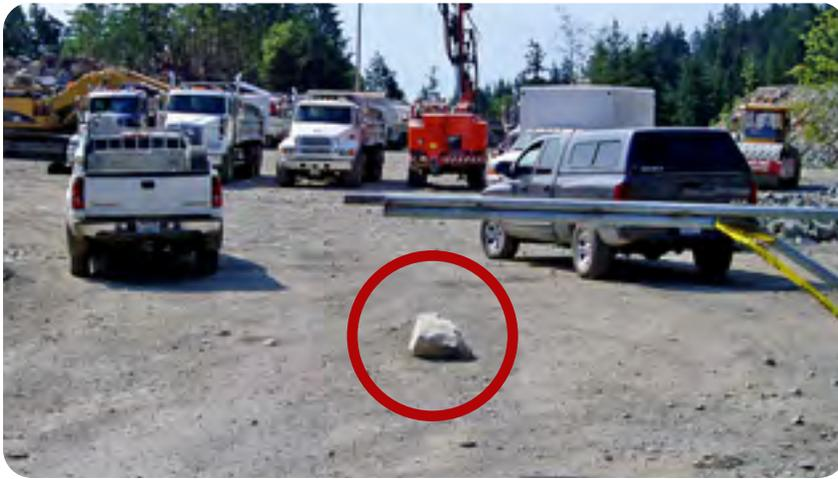
Fly rock thrown from a poorly controlled blast
