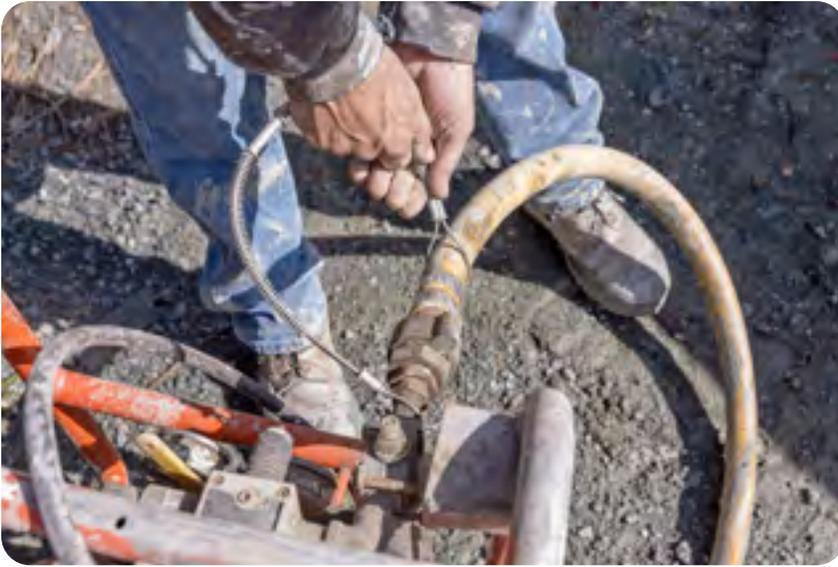
A worker installs a whipcheck (safety cable) on a compressed-air hose.
