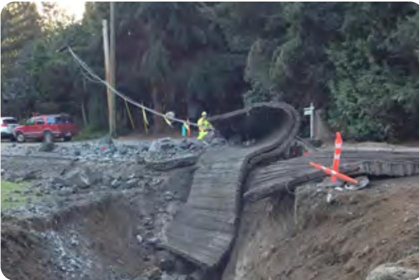
The aftermath of a blast gone wrong. In this case, the blast sent a blasting mat through the air, where it struck and brought down a power line. The blast also produced a large amount of fly rock.
