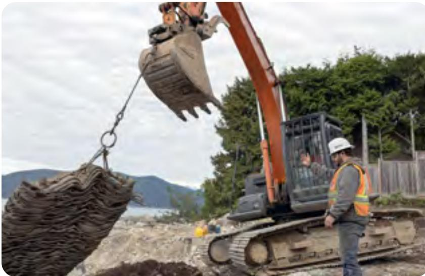
A blaster uses hand signals to communicate with a machine operator during placement of a blasting mat.
