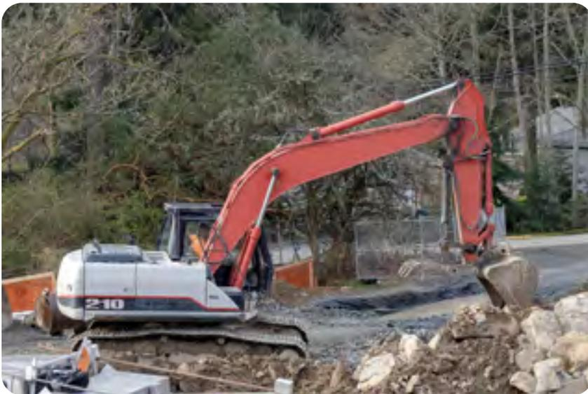
An equipment operator excavates blast rock.
