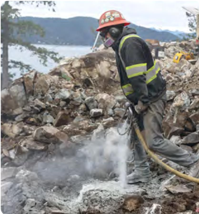
Hand-operated pneumatic rock drills expose workers to high levels of hand-arm vibration or whole-body vibration, depending on how the drill is handled.
